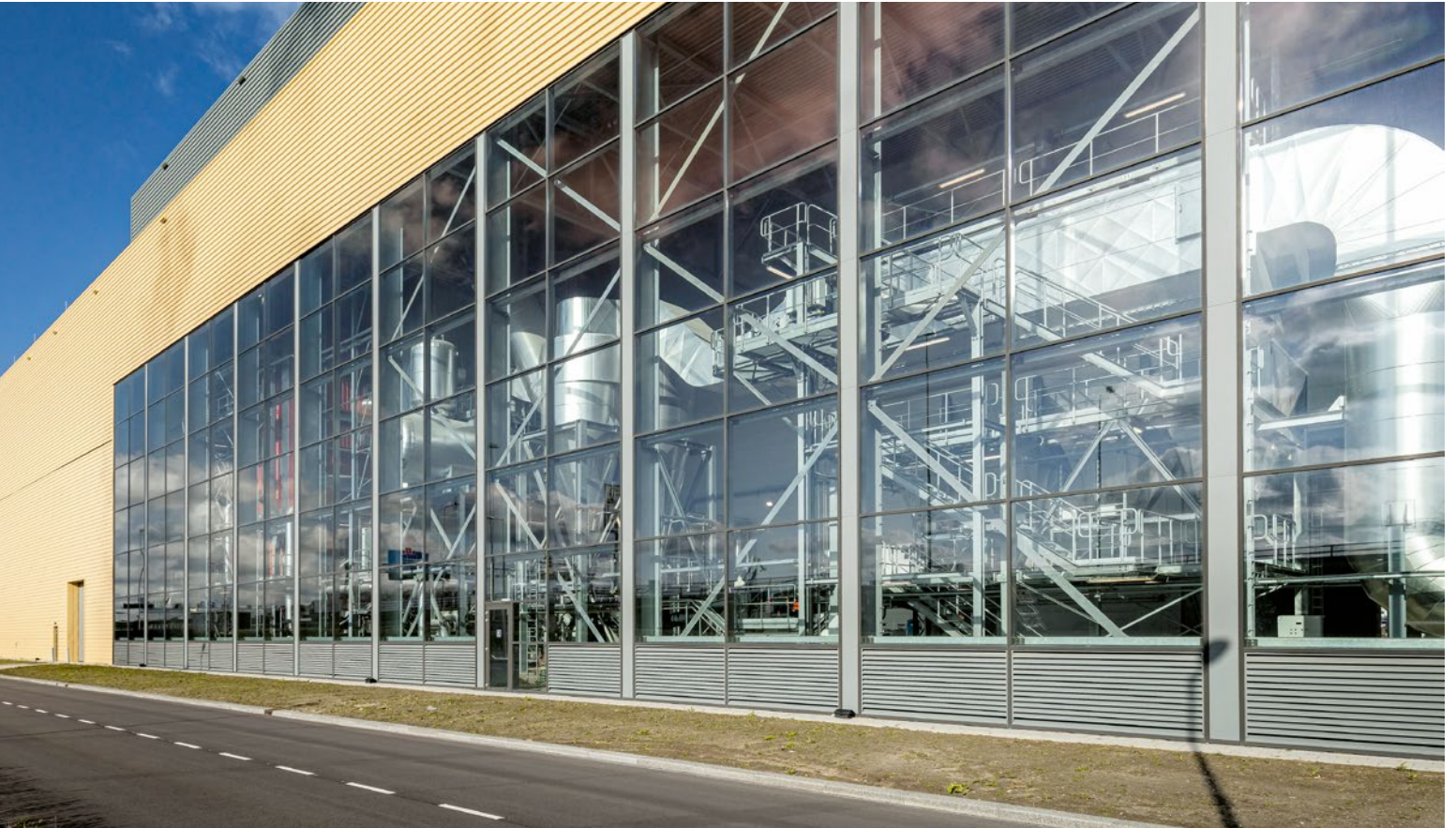
The biomass-fueled Vyncke power plant in the Netherlands.
